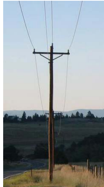
Figure 38 Three Phase Distribution
