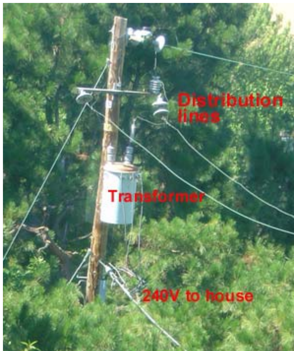
Figure 39 Transformer
