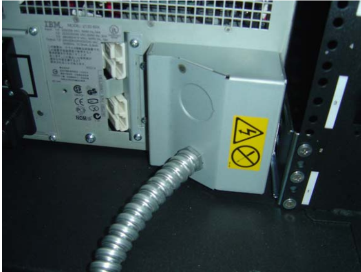
Figure 35 UPS 7500 Hardwired
