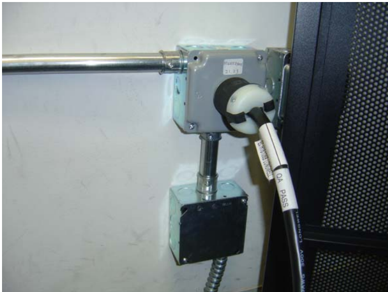
Figure 36 Hardwired Wall Connection (bottom box)
